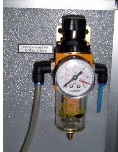
Pressure Regulator will be shipped you separately , so first you will install it the place of it as shown above left side of the machine. Two screws are provided for the installation of pressure regulator , screw them together with the pressure regulator and fix it on the left side of the machine, connect the inlet tube to the pressure regulator and connect compressed air tube (6mm) to the pressure regulator as shown shown right.
